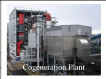
Turning heat from other process into electrical power
